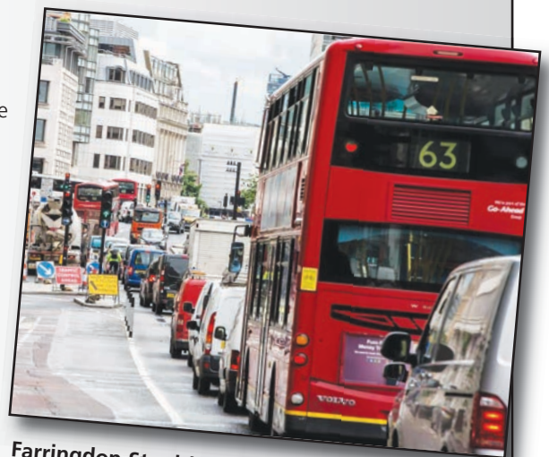
Farringdon St with Superhighway roadworks!
